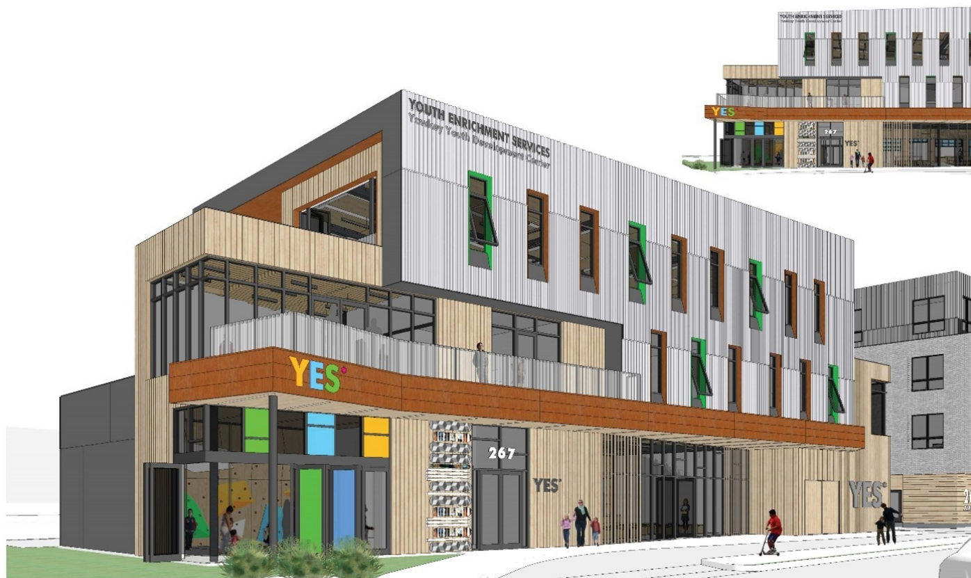
Exterior rendering of the new proposed headquarters of Youth Enrichment Services located in Jamaica Plain at 267 Amory Street. (Provided by Youth Enrichment Services)
